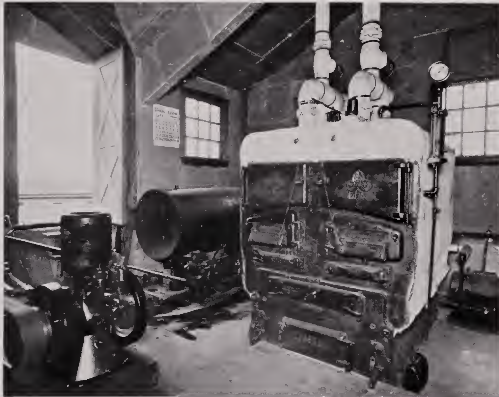
THE BOILER ROOM AND PUMP STATION
